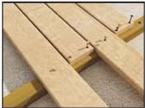
2-) Yüzeyden gizli vidalı, tapalı sistem / Stopper system hidden screwed on surface
